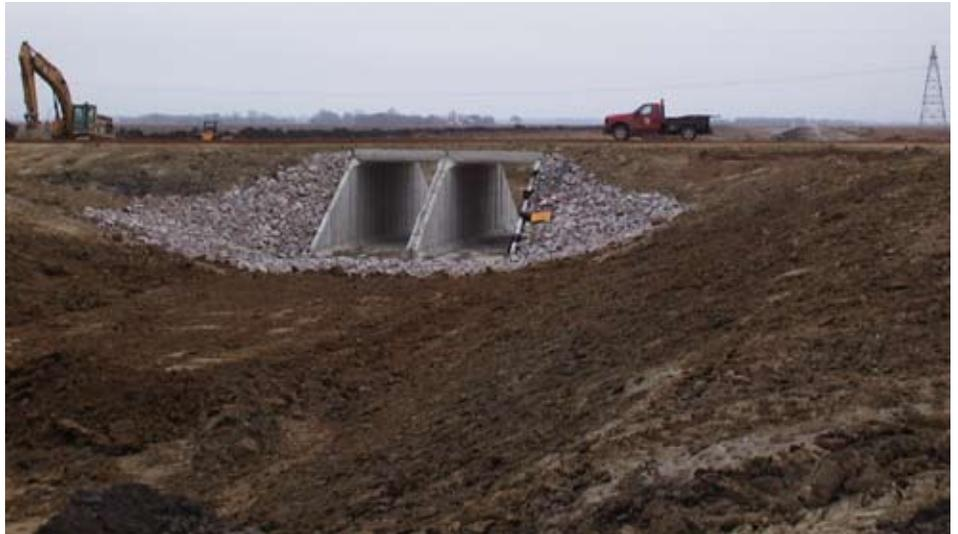
*Double box culvert under Grant County Road No. 40 on the inlet channel.*
